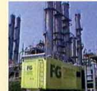
Pre-turnaround inspection on columns and structures prevent surprises during the shut-down.
