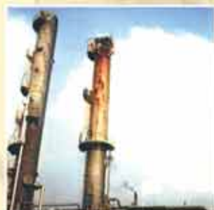
Distillation columns are inspected without erecting large scaffolding structures.
