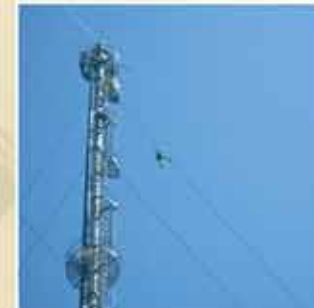
Guy-wires are inspected and coated by means of rope access.
