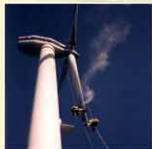
Large size windturbines are being cleaned, inspected and repaired without cranes.
